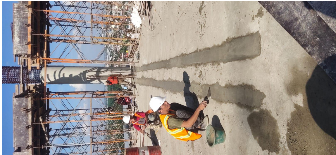
Gambar 5. Finishing pengecoran
