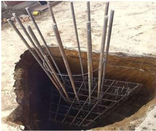
Gambar 1. Pondasi Bore Pile
