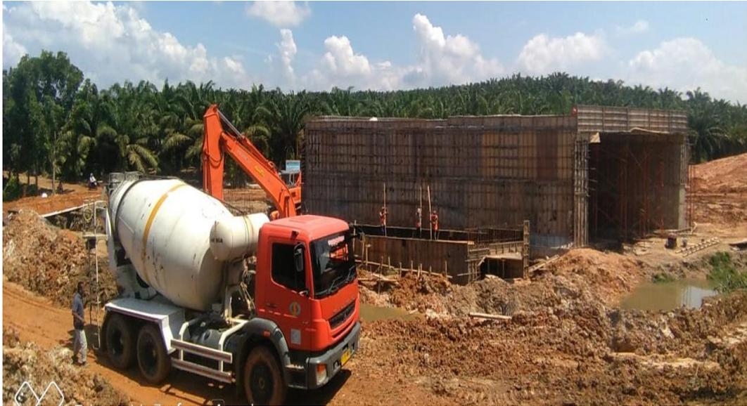
*Gambar 2.5 Underpass Box Culvert*
