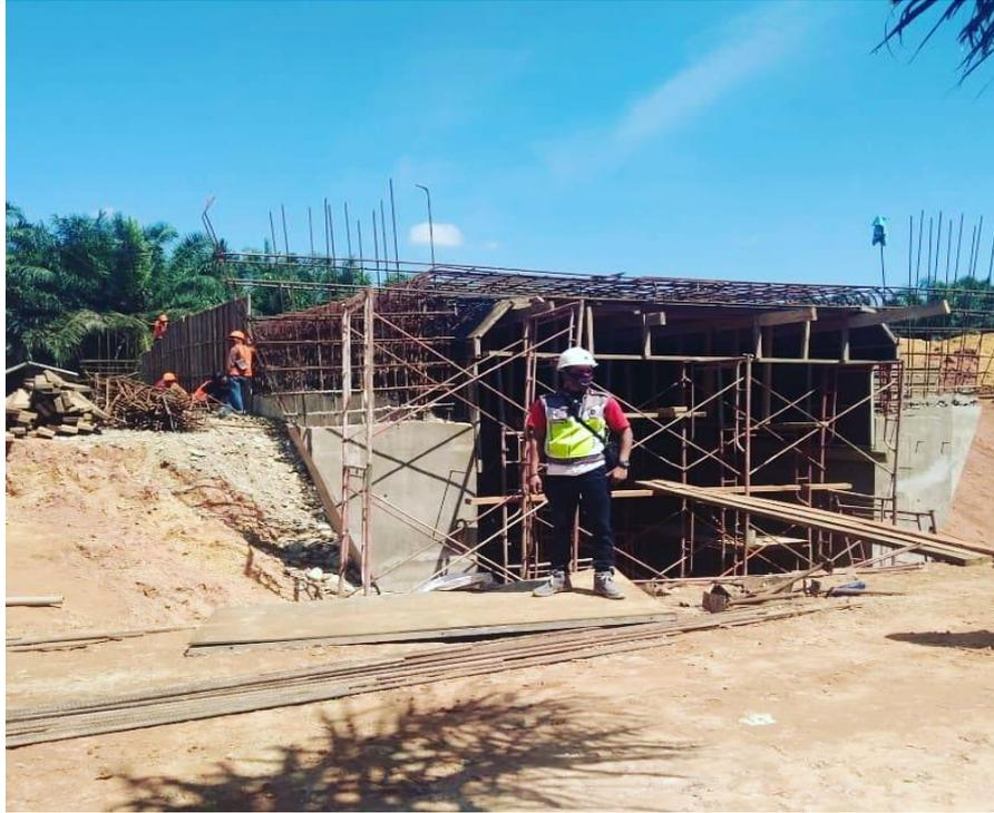
*Gambar 2.7 Underpass Box Culvert*
