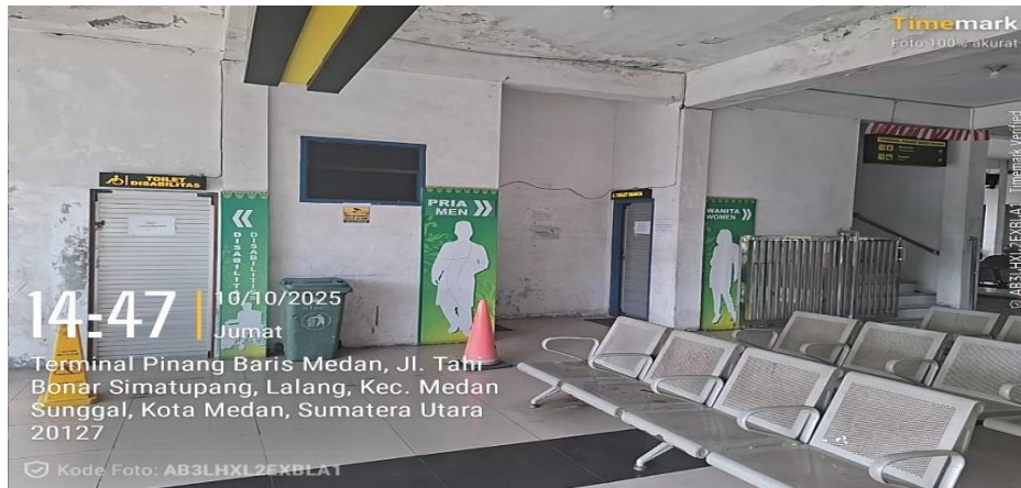
Lampiran 12. Gambar Fasilitas Toilet Terminal
